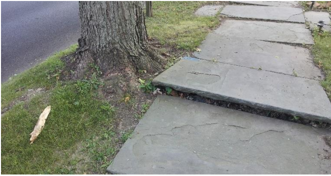
Tree roots heaving pavement
