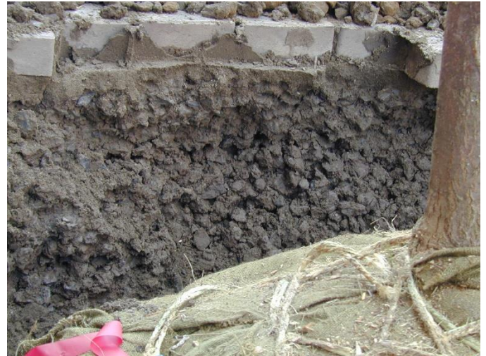
Closeup of CU-Structural Soil® after installation
