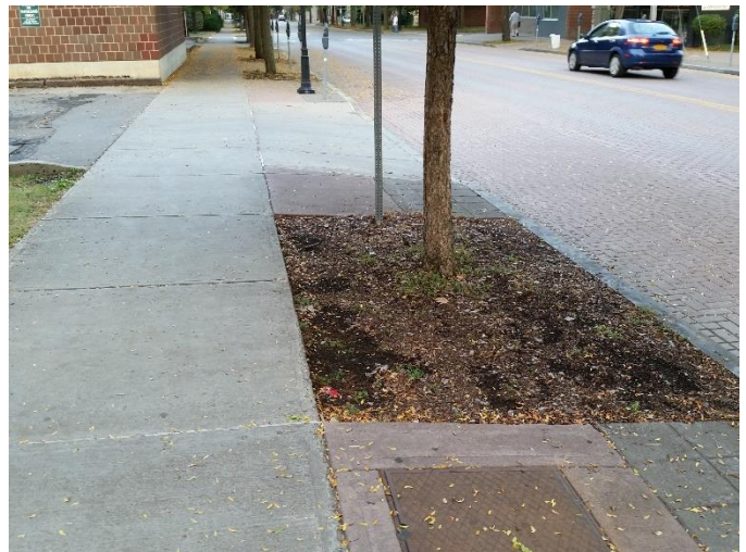
A typical tree pit on W. State Street. The colored concrete sections correspond with the extents of the CU-Soil® volume.
